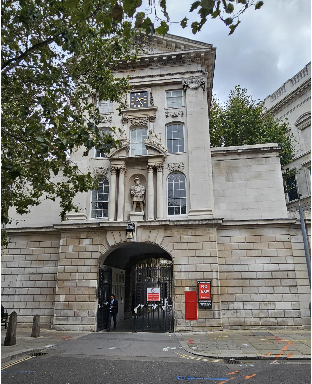
Restoration of Henry VIII's Gate delayed Phase 2 works, West Smithfield/Giltspur Street
