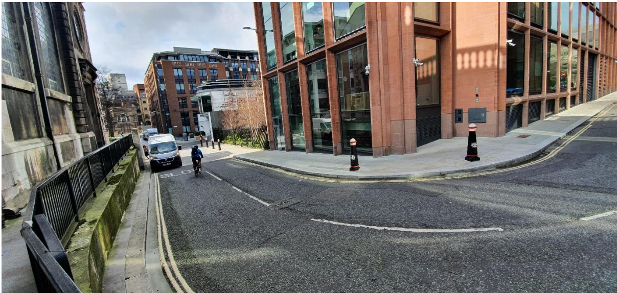
Distaff Lane footway around 2-6 Cannon Street development | Completed
